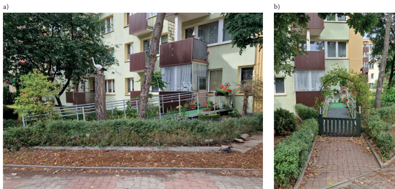
Figure 4. Proper example of ramp access to a balcony in a multi-family building: a) side view showing height difference to first floor level and the entrance to the balcony, b) closing gate to the ramp, 2025, Białystok, Poland
